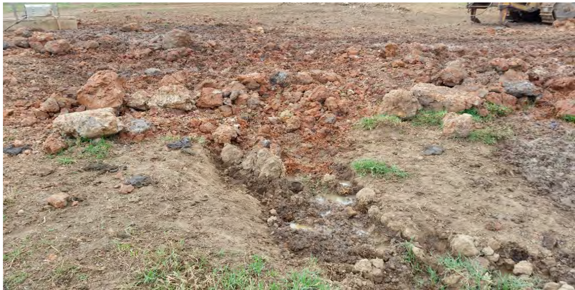
Photograph 6 - View north toward Area B filling
