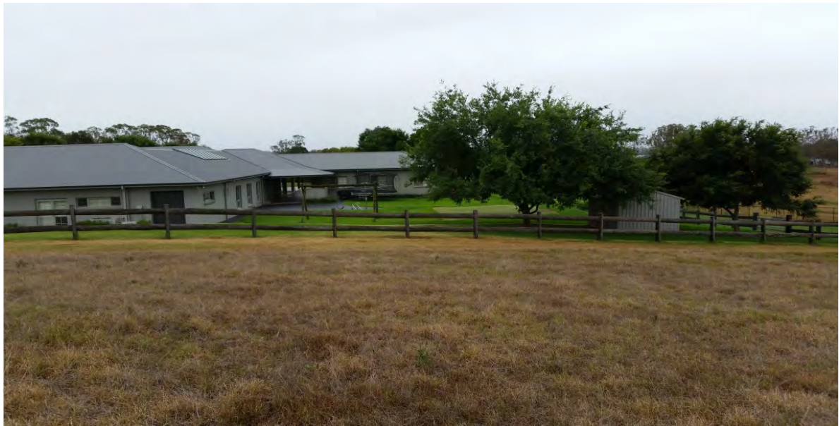
Photograph 1 - View facing north towards residential property 1
