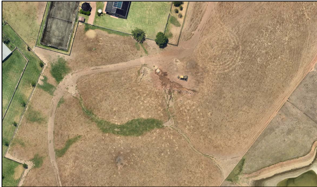
Figure 1: Nearmap image (23 January 2017) showing filled drainage channel and the access road.
